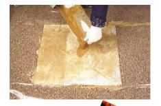
This was the perfect solution for bridging the gap inside the interceptor, but we had to consider the void space within this area as the packer would also expand to this profile which could possibly burst the packer and result in a defective NO-DIG solution. The solution to make sure that we protected the packer & the
